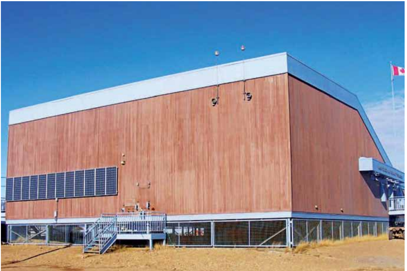
Angik School, Paulatuk, 2.1 kW Grid-tie, Installed 2011 – Photo Credit: Bart Coumont
