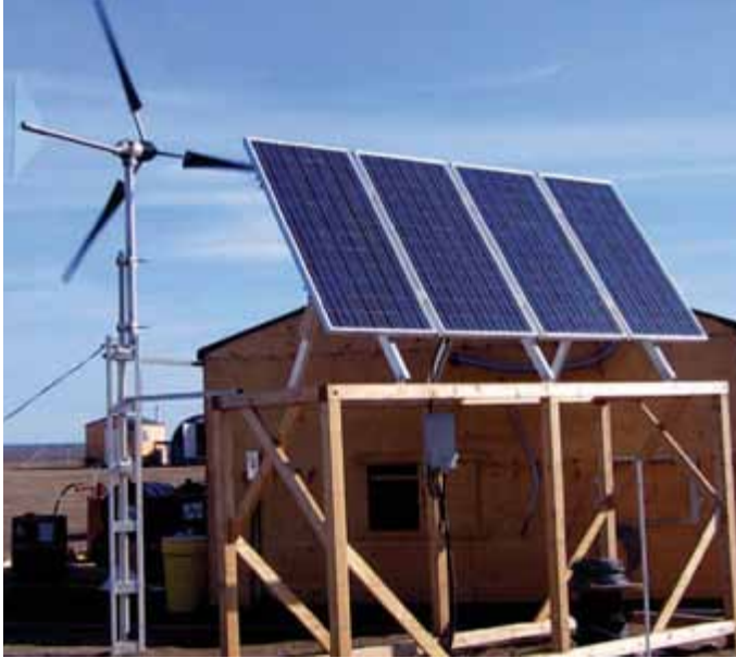
Rio Tinto Exploration Camp, Banks Island. Off-grid Battery Charging System. Installed 2011 – Photo Credit: Paul Jones
