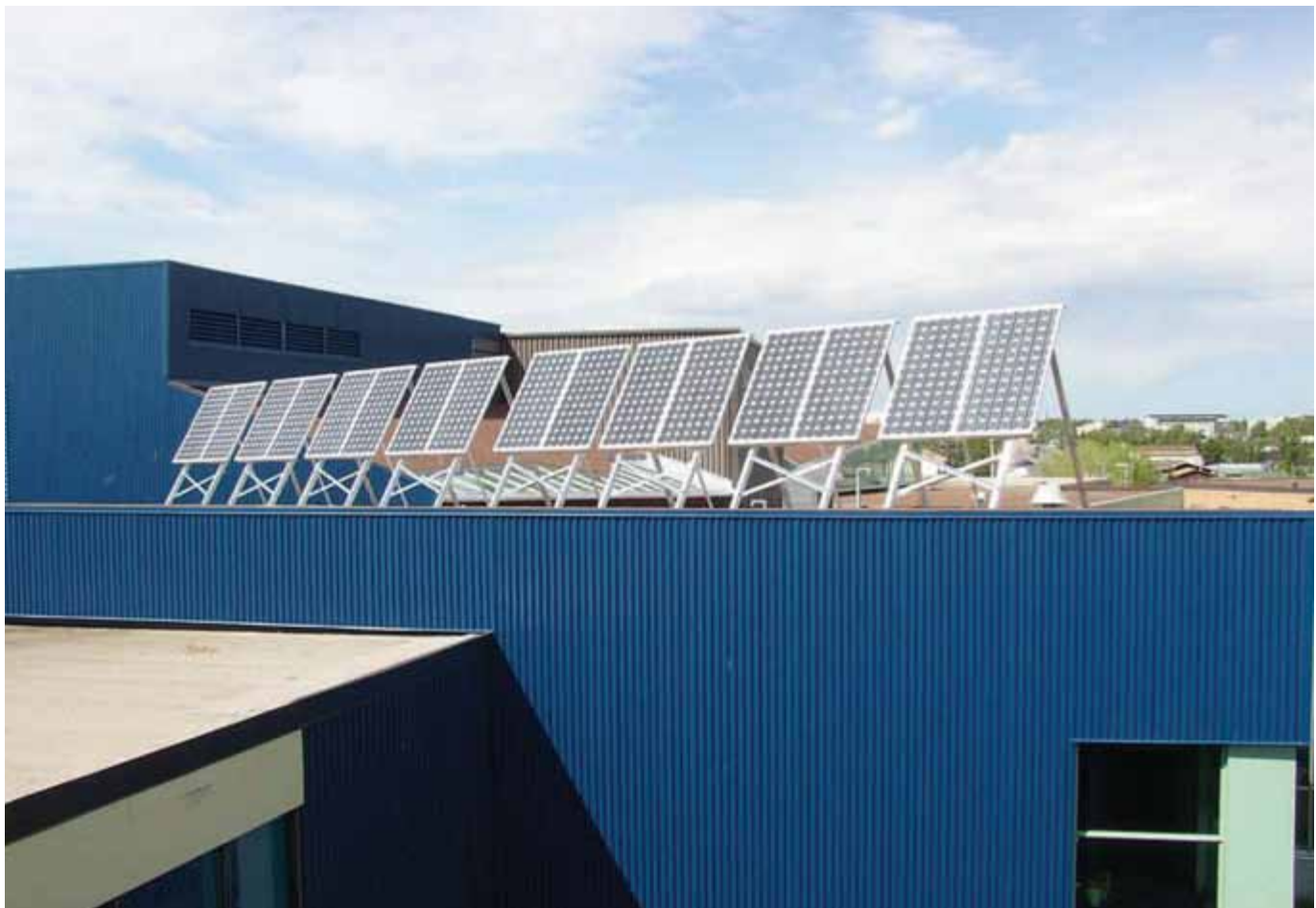
Sir John Franklin High School, 2 kW Grid Interconnected, First Public Grid-tie in the NWT, Installed 2003 – Photo Credit: Wade Carpenter
