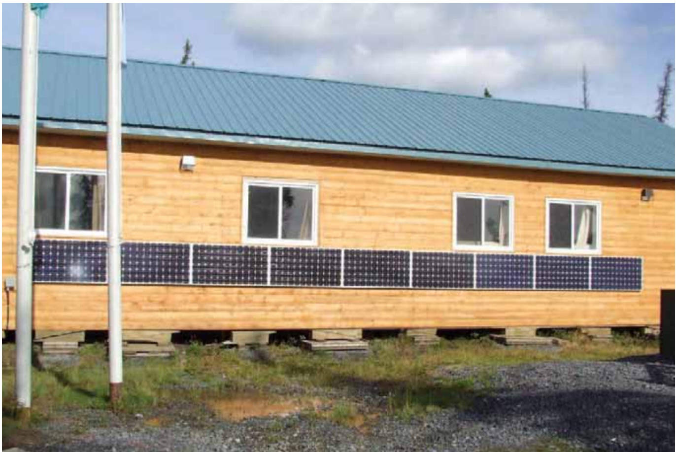
Gwich'in Wellness Camp, 1.7 kW Isolated Diesel Grid Interconnection, Installed 2010 – Photo Credit: Matthew Brost
