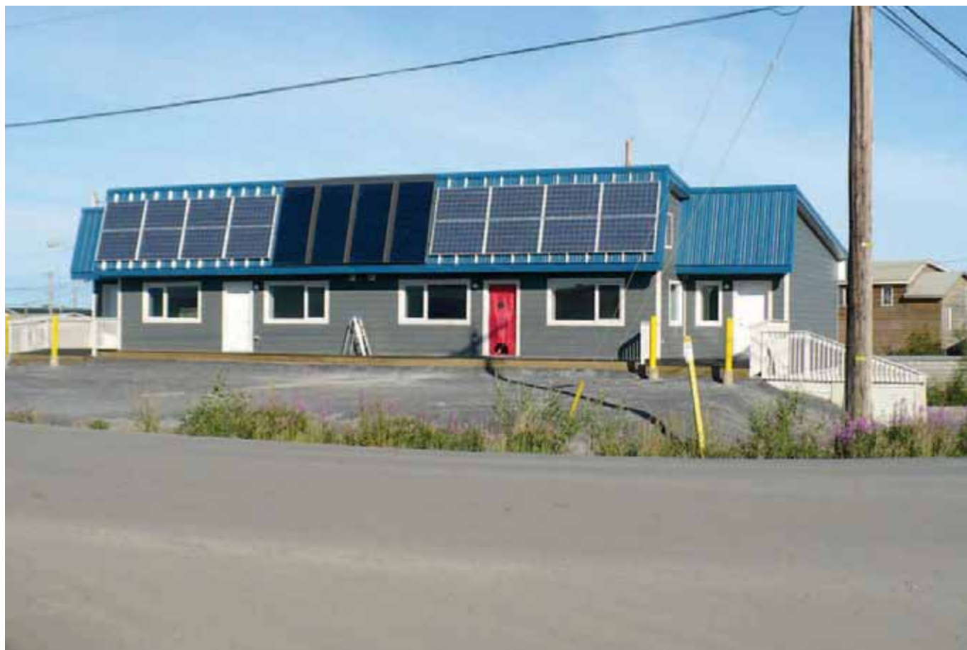
Northern Sustainable Housing Project, Inuvik, Solar PV and Solar Hot Water, Installed 2012 – Photo Credit: Wade Carpenter/GNWT
